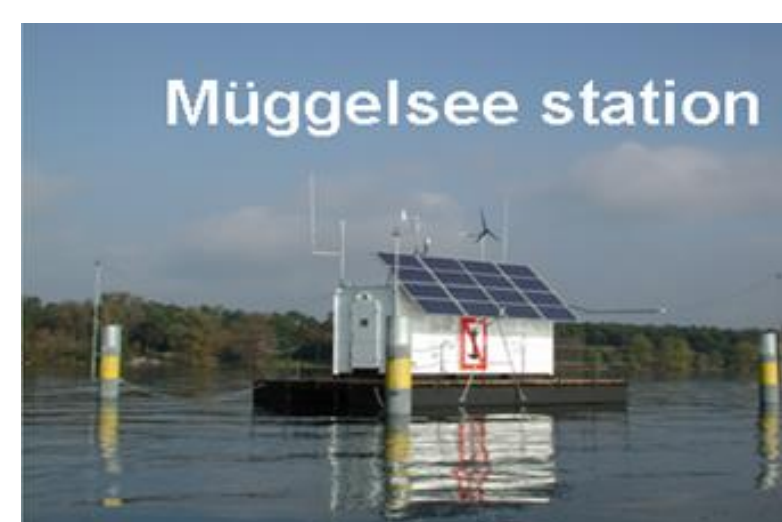
Automatic in situ measurements
